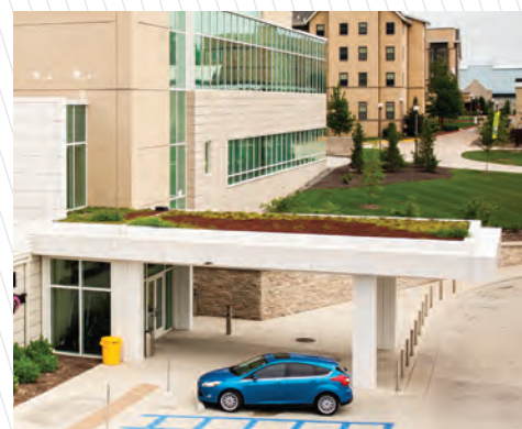
Green Roof at Patient Care Tower. Reduces and slows stormwater runoff.
