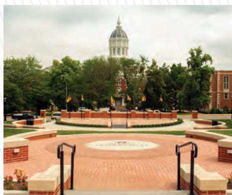
Pervious Pavement at Traditions Plaza. Filters pollutants and reduces runoff.
