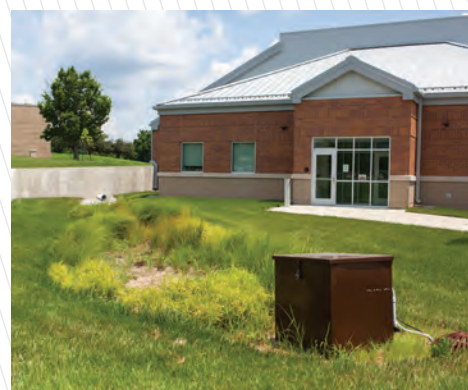
Bioretention at Animal Resource Center. Reduces runoff by pooling and filtering excess water.
