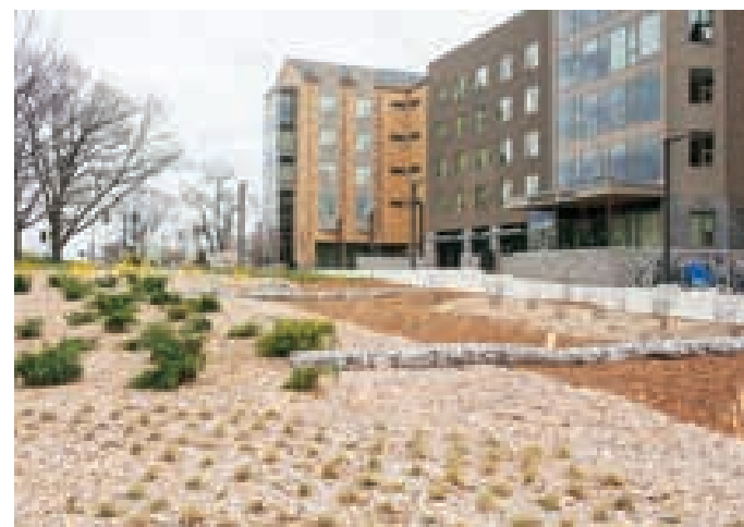
A bioswale outside of Gateway Residence Hall filters and reduces stormwater runoff and pollution.
