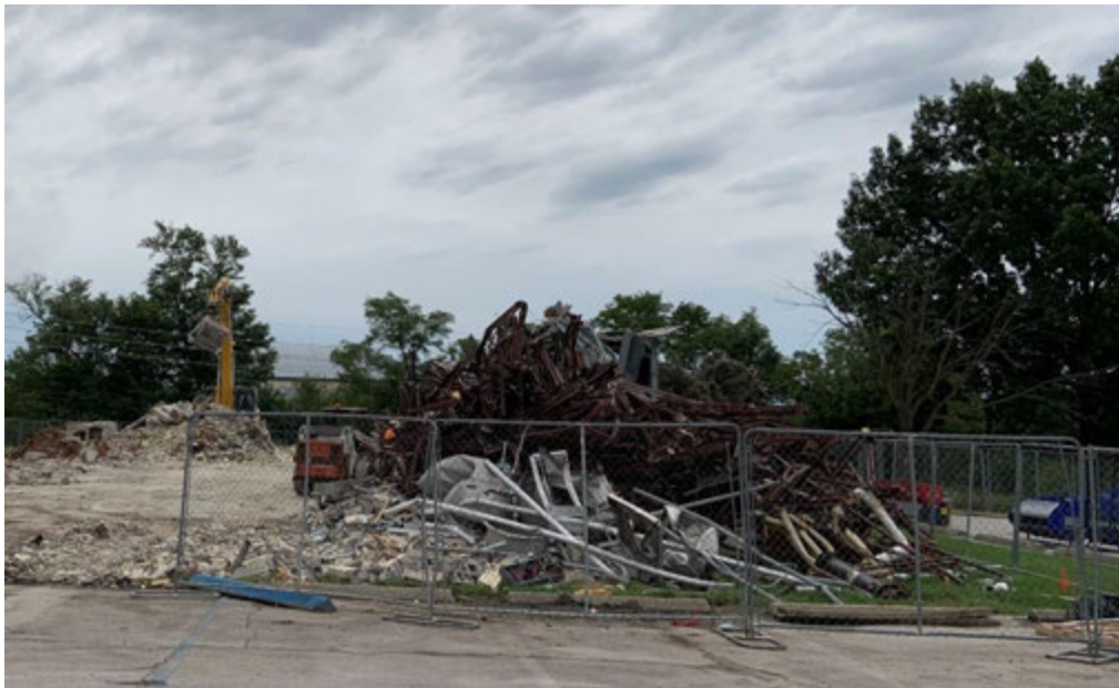
(Photos above): Demolition of the Research Park Development Building
