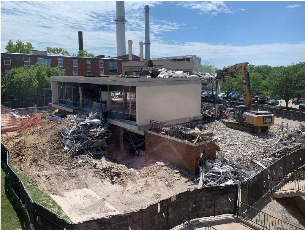
Loeb Hall Demolition
