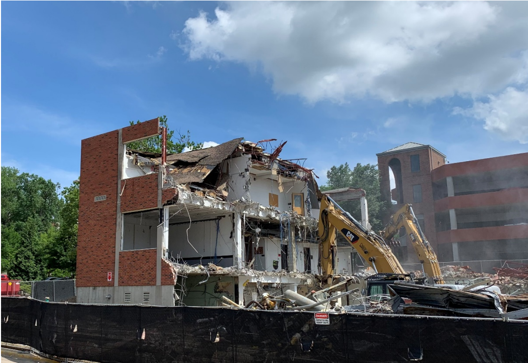
London Hall Demolition
